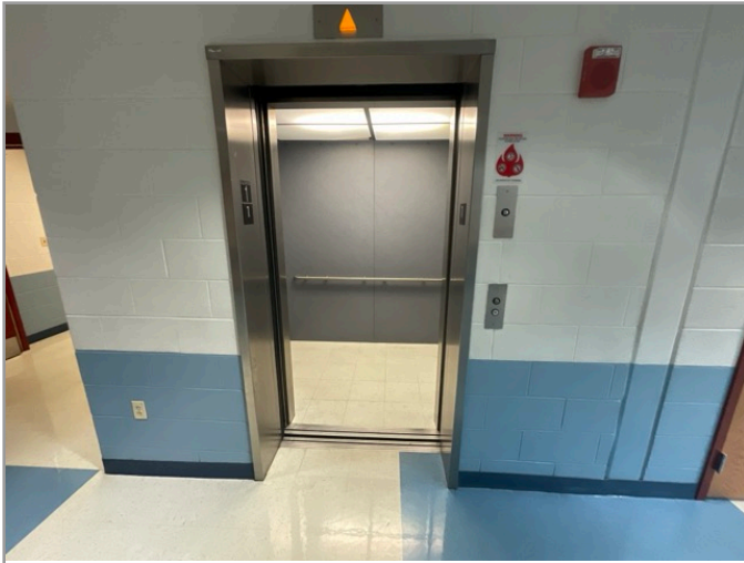
LOBBY LOOKING AT CABS
