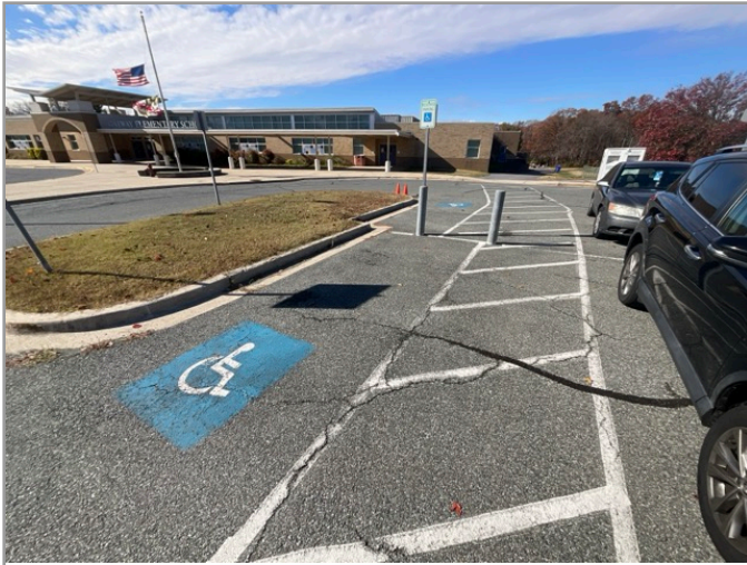
OVERVIEW OF ACCESSIBLE PARKING AREA
