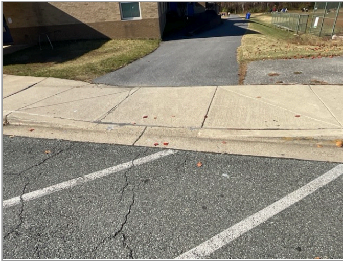
ACCESSIBLE ROUTE TO PLAYGROUND
